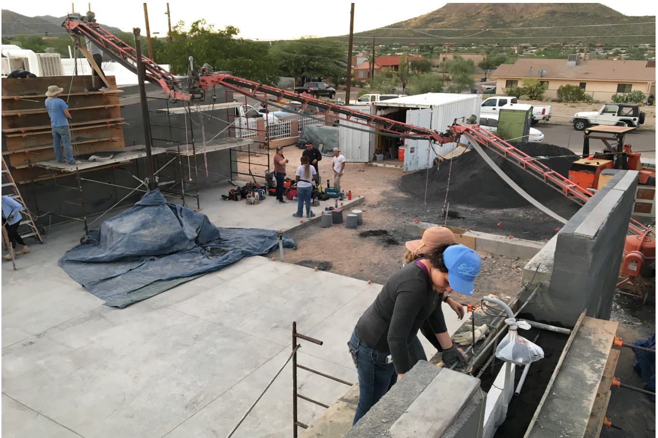
Figure 6. Students construct scoria walls. Photo by Queston Kwolek.
