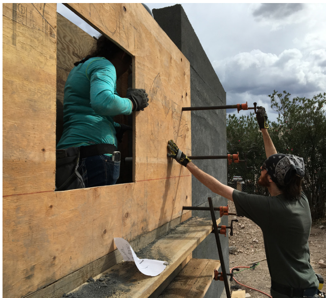
Figure 7. Formwork for window box. Photo by Queston Kwolek.
